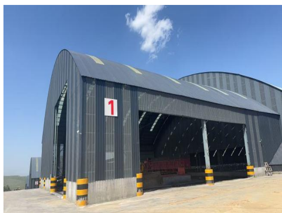
1#全封闭卸煤棚
